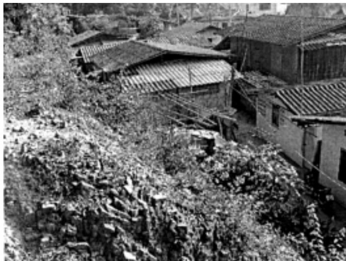
Figure 4. The earthen wall after the houses have been moved.
