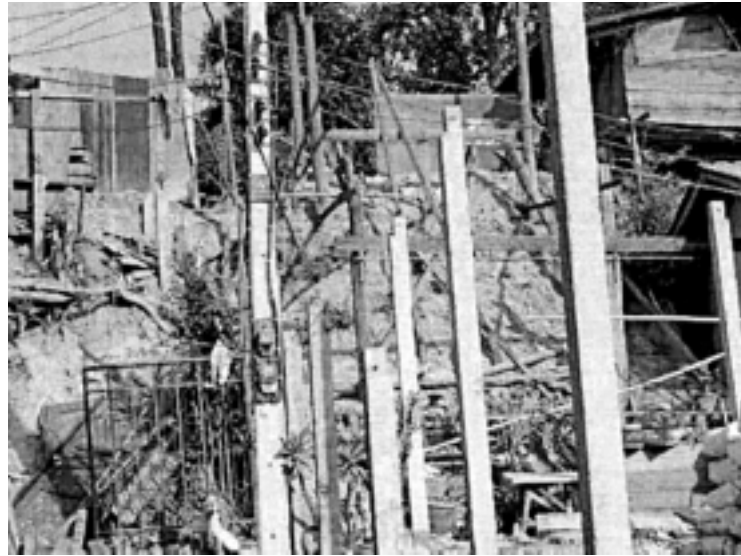
Figure 3. The construction of houses that move to resettle on the land.
