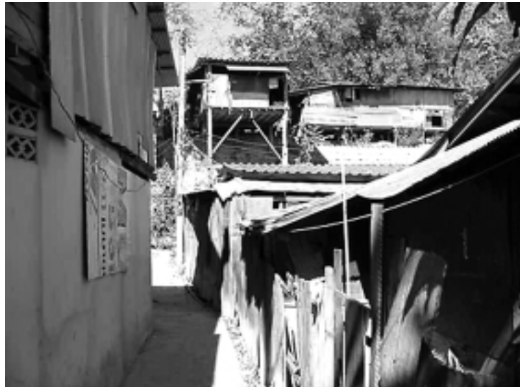
Figure 2. The invading houses on the remnant of the historical earthen wall.
