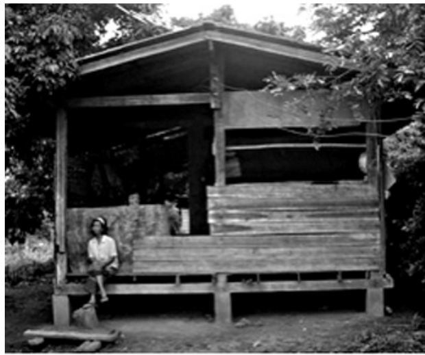
Figure 1. Due to rare wood resource, repairing by timber is expensive for the low-income villagers.
