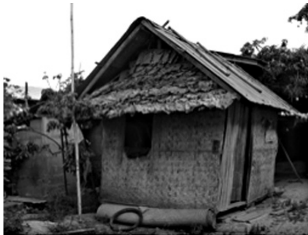
Figure 2. Variety of construction wall materials of typical low-income housing.
