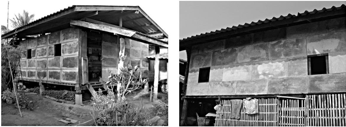
Figure 8. Repaired houses by this natural-fiber cement board technology.
